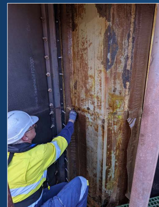
Removal and inspection
